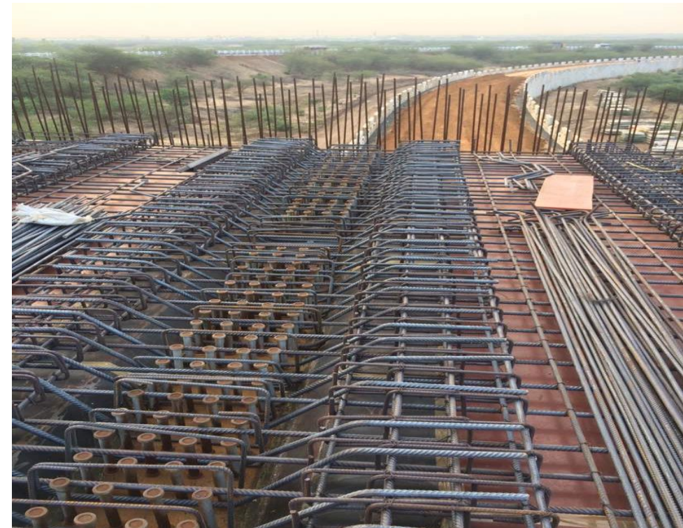
Flyover in Madurai - Ramanathpuram Section
