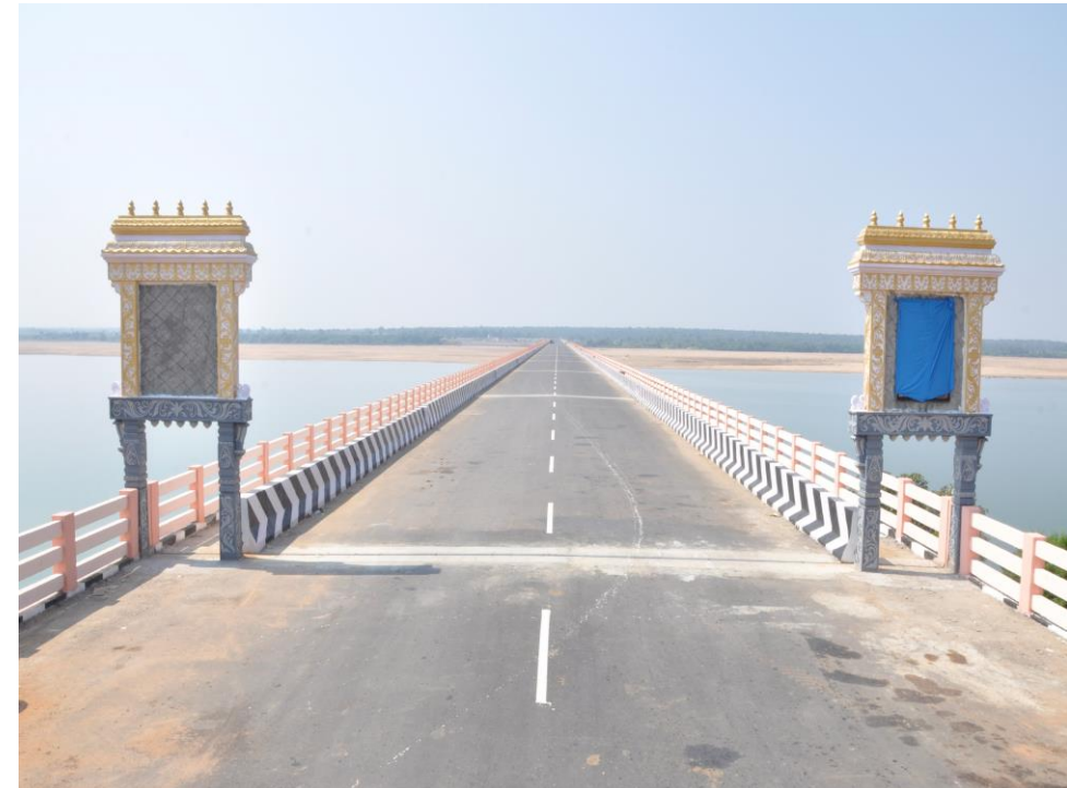
Eturunagaram Bridge over river Godavari
