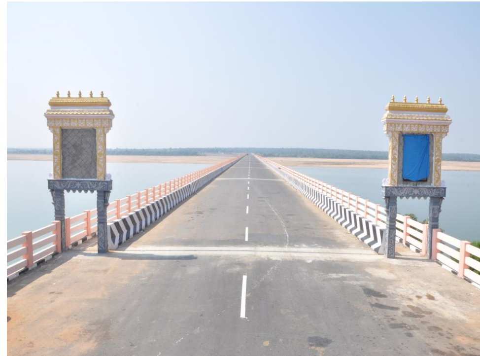
Eturunagaram Bridge over river Godavari
