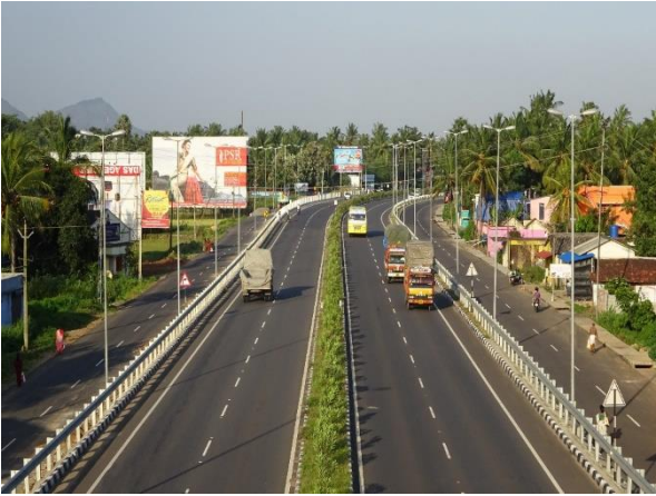
Walayar Road Project
