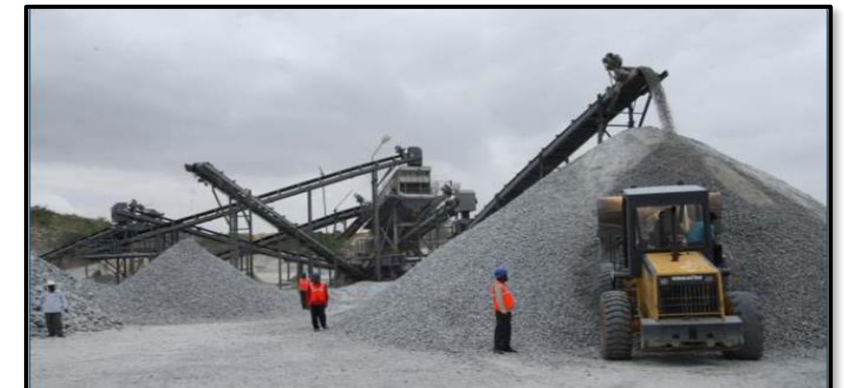
250 TPH Nawa Crushing Plant
