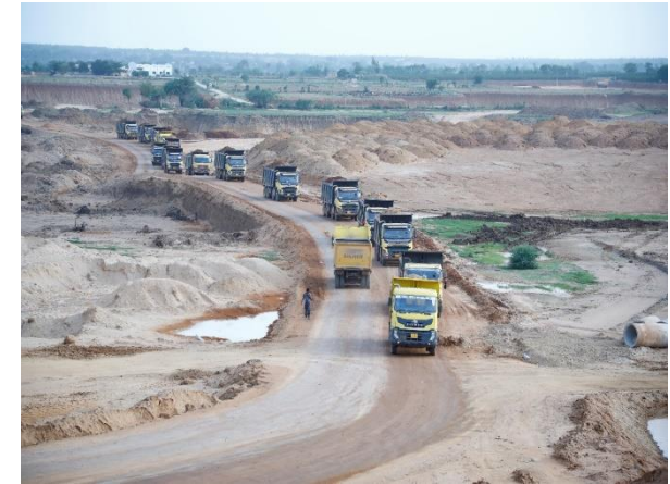
Tippers at Irrigation Site
