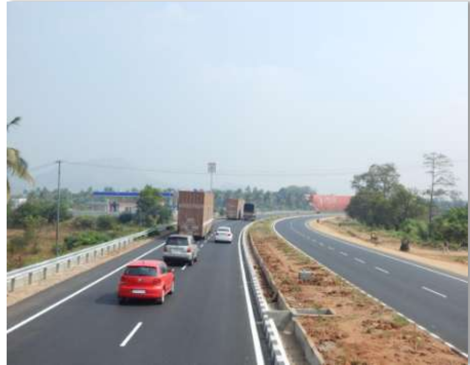
Walayar –Vadakkancherry BOT (Toll Road ) Project, Kerala
