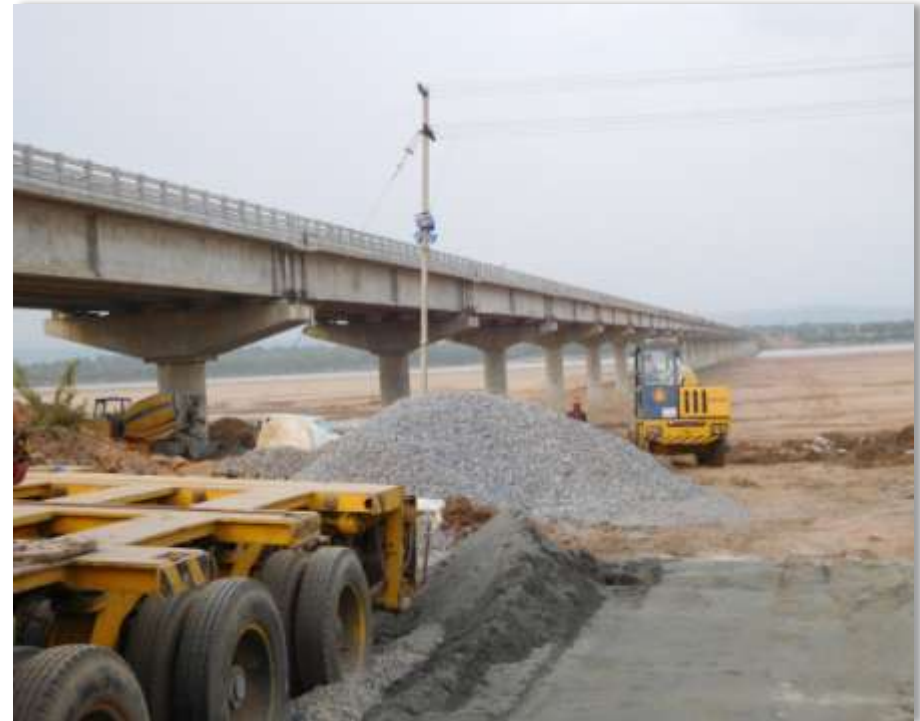
Bridge across River Godavari in Telangana State
