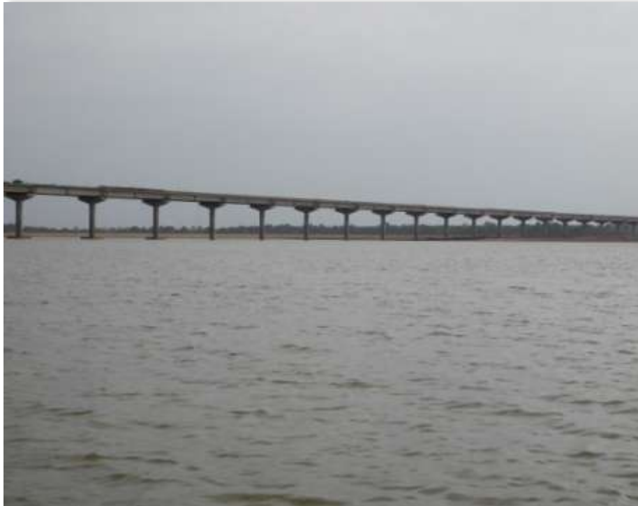
Bridge across River Godavari in Telangana State
