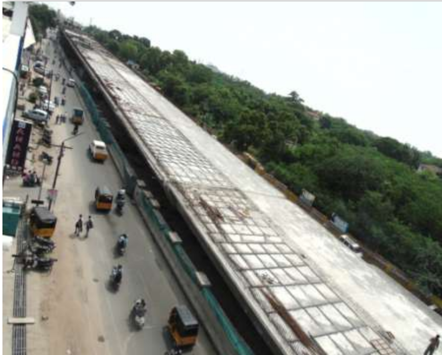
Flyover at Coimbatore in the State of Tamil Nadu
