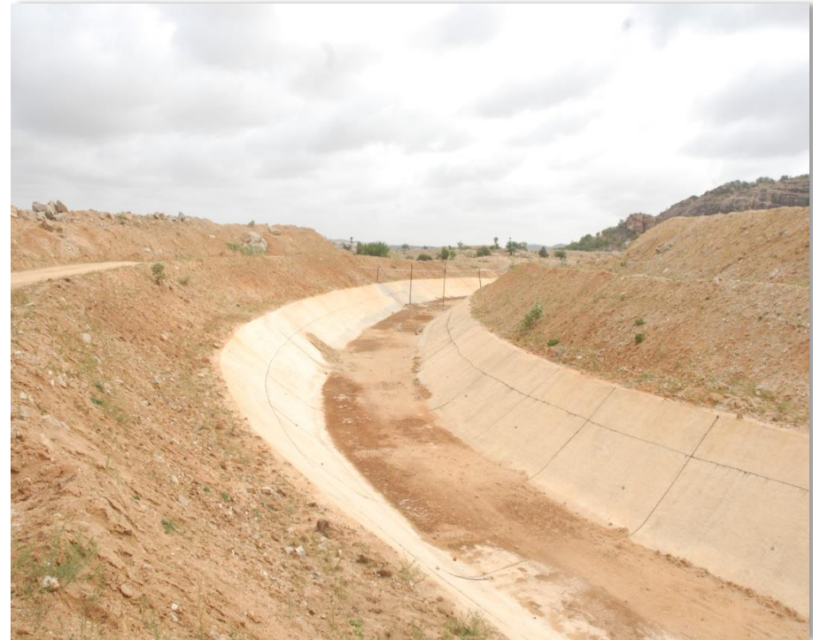
Irrigation Project in Telangana State
