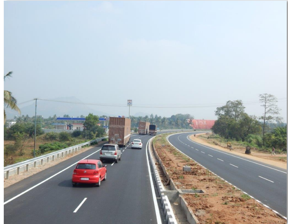
Walayar –Vadakkancherry BOT (Toll Road ) Project, Kerala
