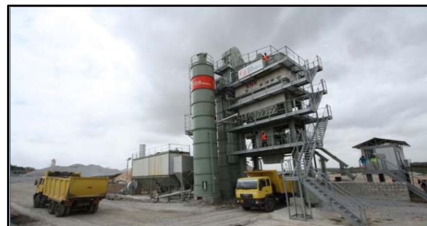
240 TPH D & G Hot Mix Plant
