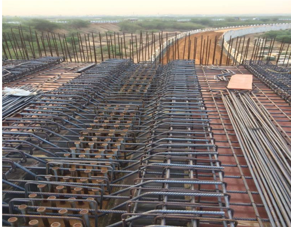
Flyover in Madurai - Ramanathpuram Section
