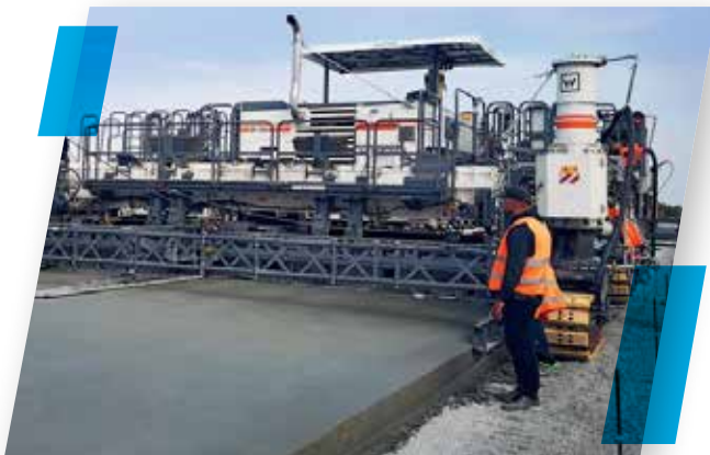
WIRTGEN SP1200 PQC SLIPFORM PAVER
