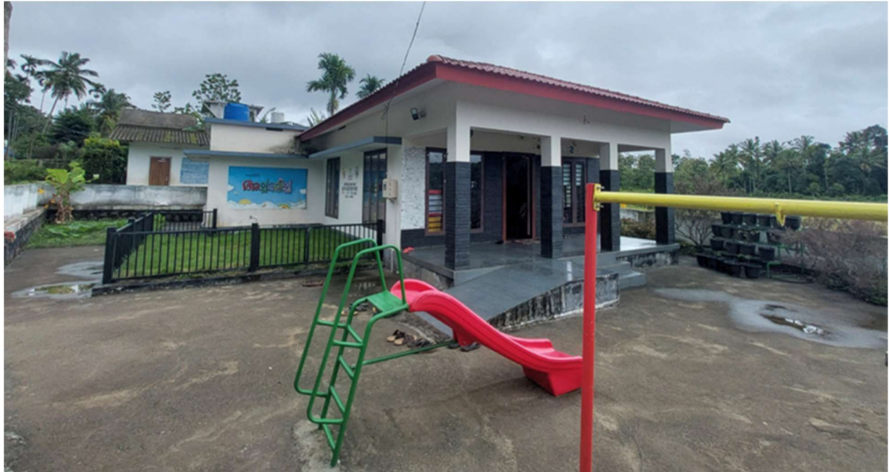
Pic 3 – Overview of the newly constructed Anganwadi centre.
