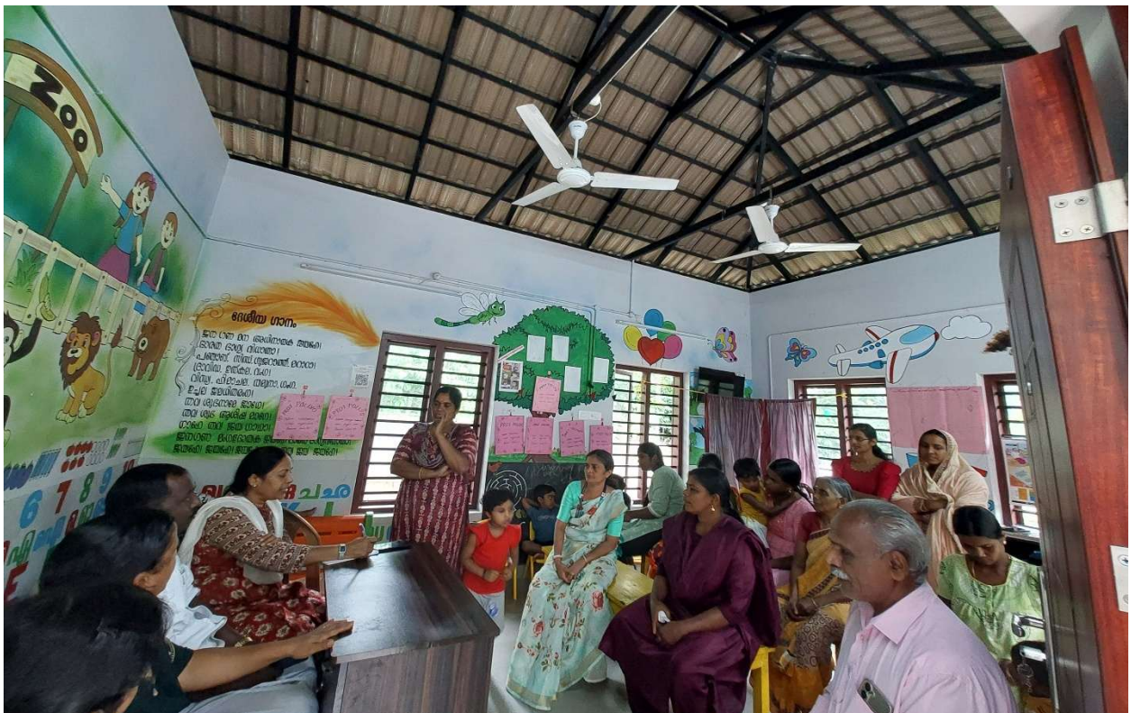
Pic 6 - Interior view of the Anganwadi centre highlighting the roof structure, thematic wall paintings, and stakeholder interaction.
