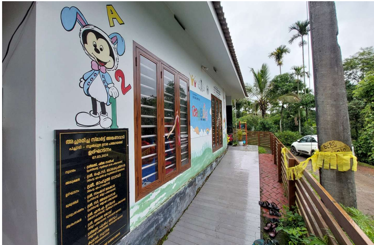
Pic 12 – Lateral view of the Anganwadi centre showing the side pathway and wide windows for natural ventilation.
