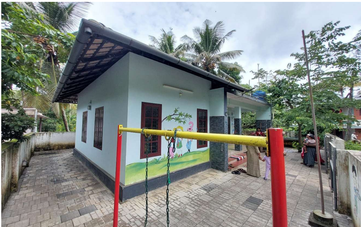
Pic 2 – Angular view of the newly constructed centre with spacious outdoor surroundings.
