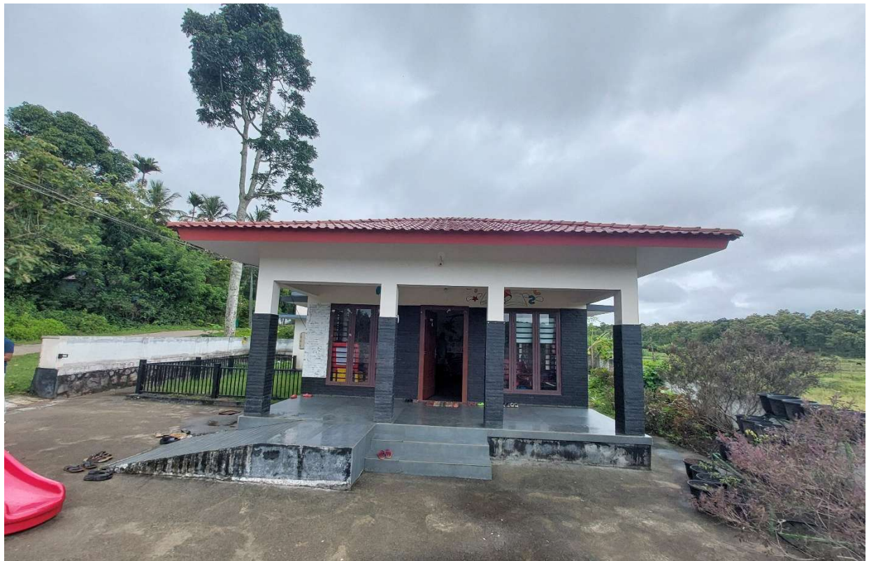
Pic 4 – Newly constructed Anganwadi centre showing the inclusive design with a ramp and steps, spacious outside area, and space for nutrition garden.
