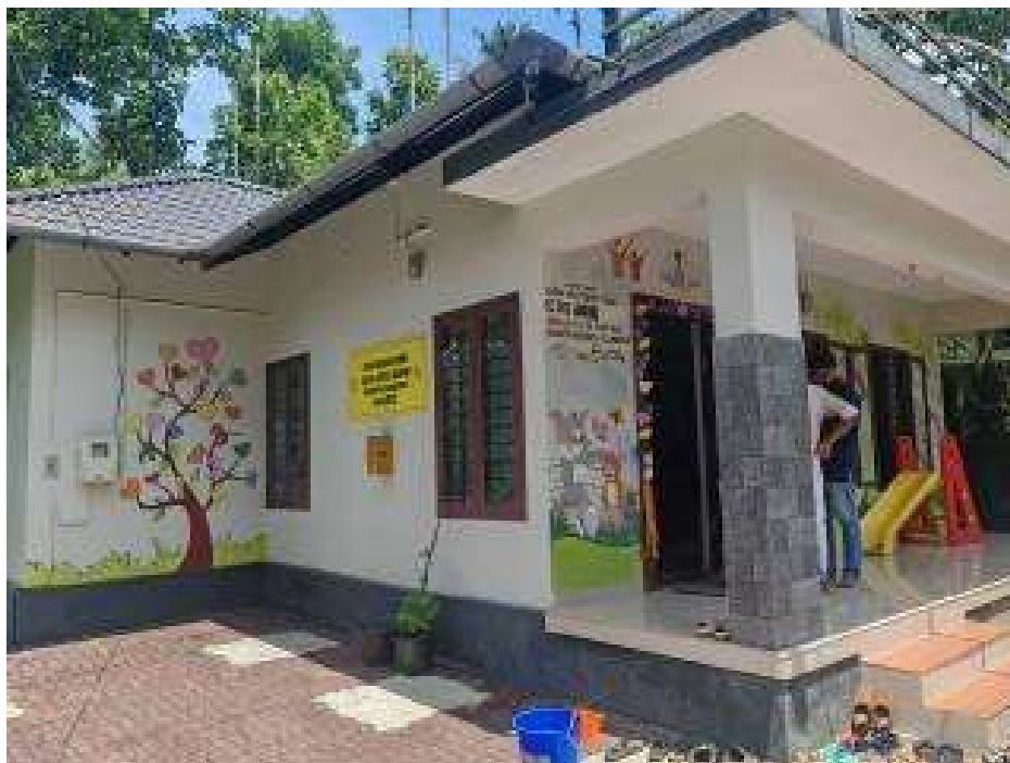
Pic 13 – Corner view of the Anganwadi centre with ample open space for children's outdoor activities.
