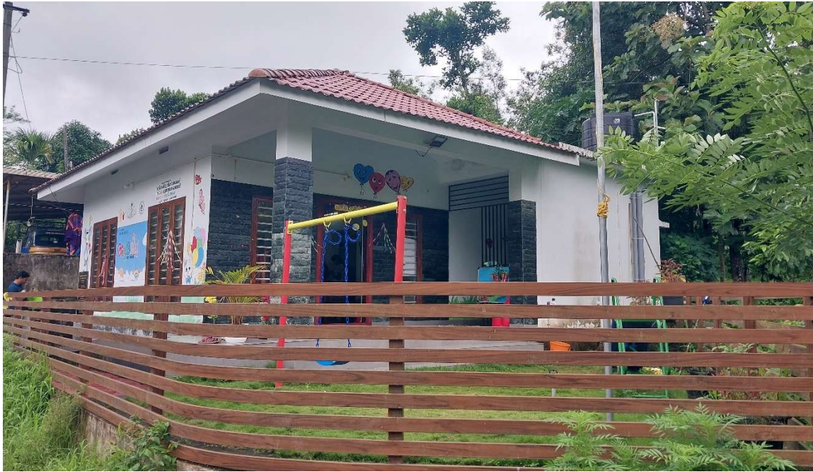
Pic 1 – Newly constructed Anganwadi centre with a secure iron fence and gate.
