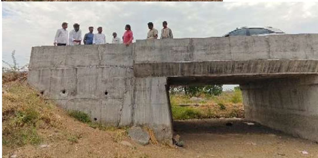
Pic 12 – Assessment team observing the slab culvert, highlighting the opening and abutments.
