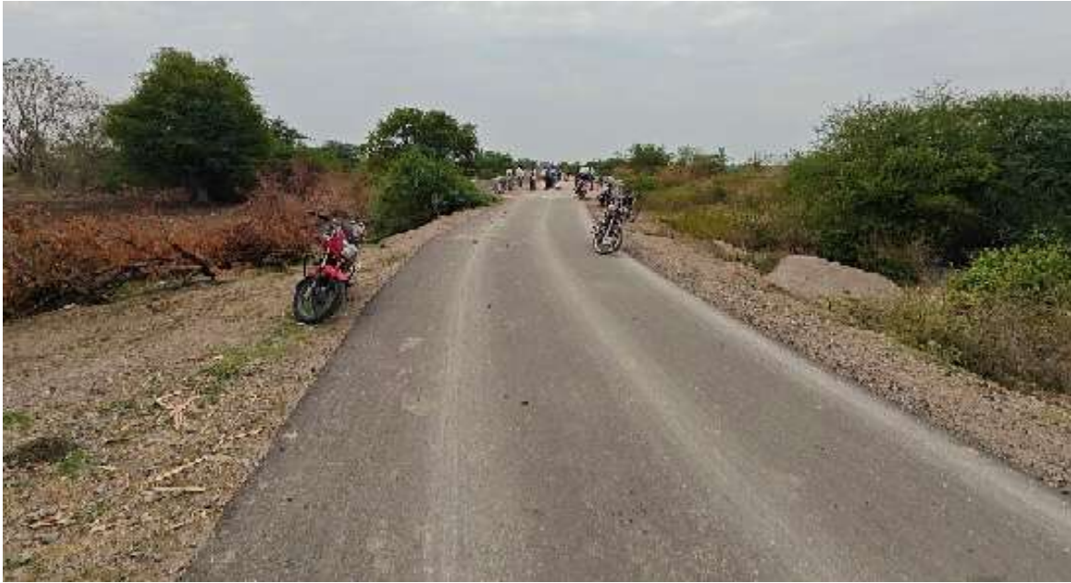
Pic 5 – BT road featuring extended shoulders for improved safety and durability.
