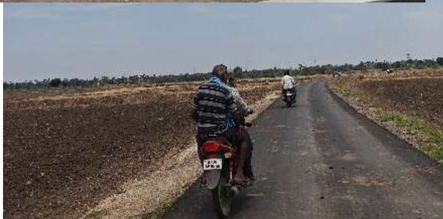
Pic 6 & 7 – Villagers using the newly constructed road for their everyday activities.
