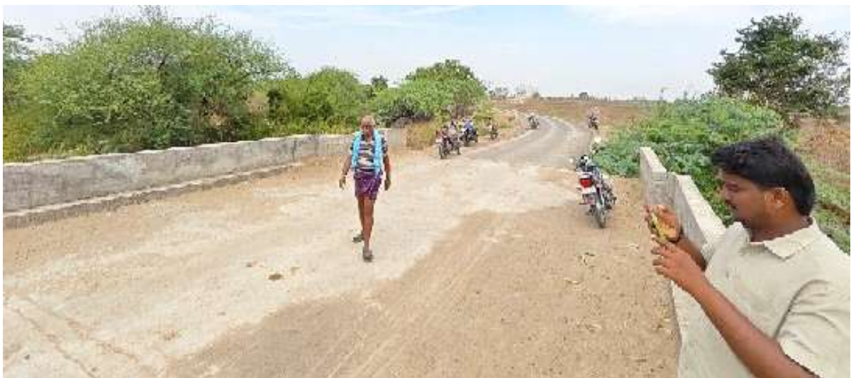
Pic 8, 9 &10 – Well-constructed slab culverts built to prescribed quality standards.
