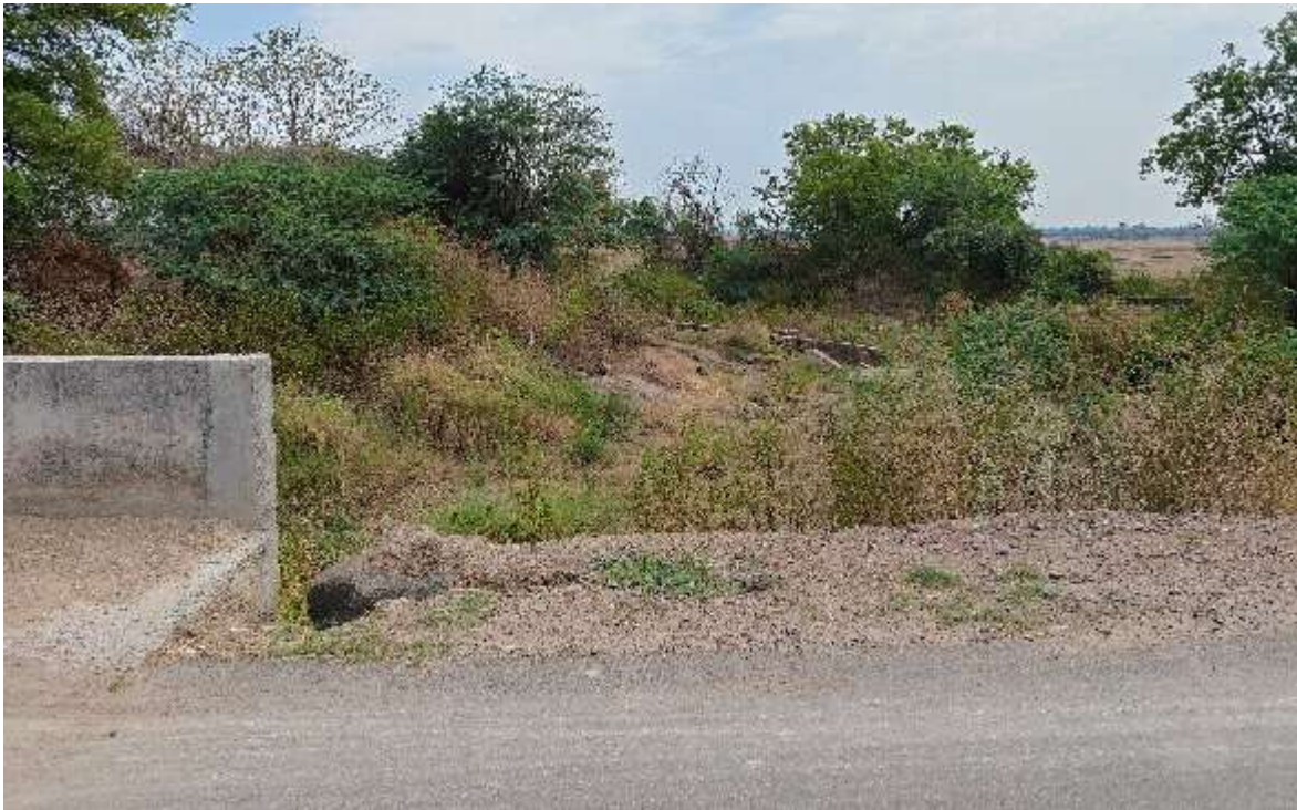
Pic 17 – View of the natural stream channel conveying stormwater to the culvert.
