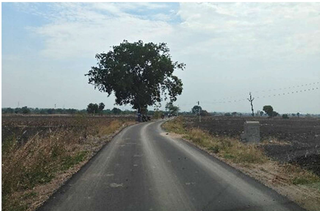
Pic 1 & 2 – Black Top road constructed to enhance access to agricultural lands
