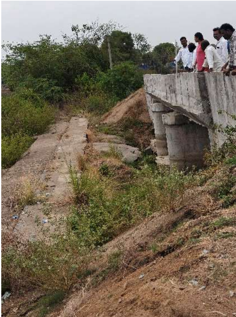
Pic 11 – View of the slab culvert showing the footings, bed protection, slope protection, and parapet wall.
