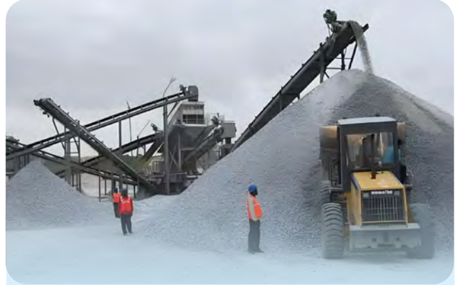
250 TPH Nawa Crushing Plant
