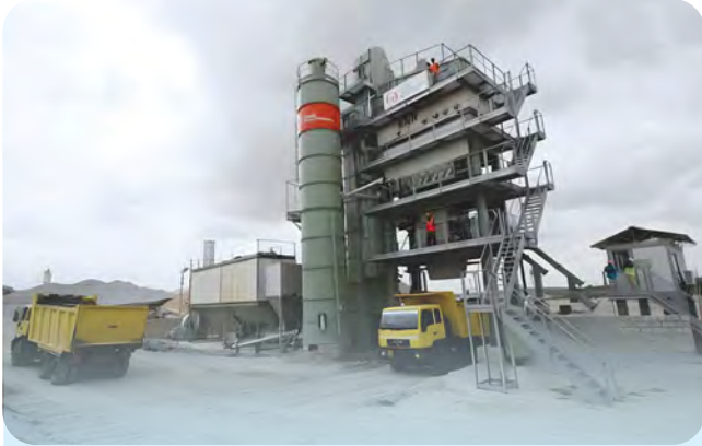
240 TPH D & G Hot Mix Plant
